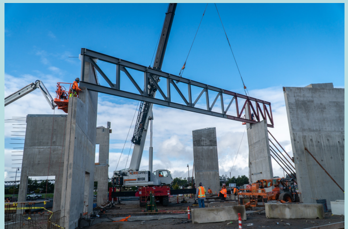
Construction of the new Marine Studies Building. c/o Mark Farley
